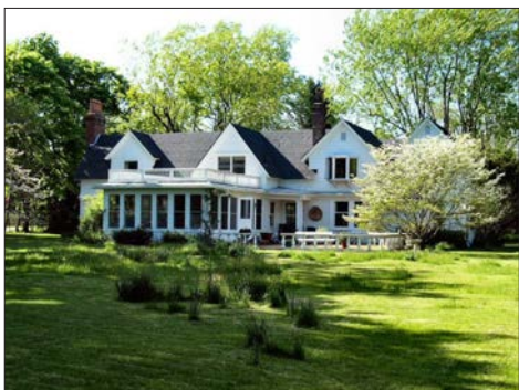
Fire Place Farm, built mid-19th Century onward. View is from the back looking north.
