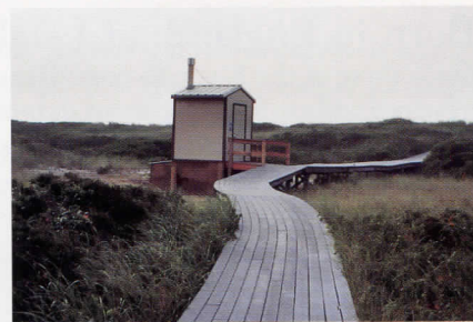
Photo courtesy of Jeb Barry
