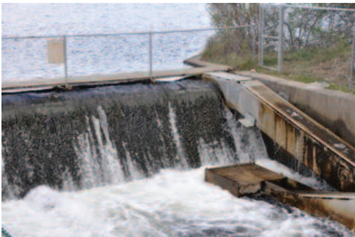
10 – Fish ladder at Sunrise Highway.
