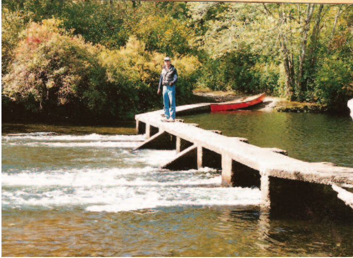
16 – Mid River Dam in Southaven Park.
