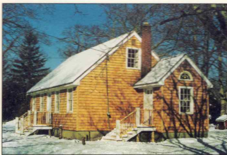
The newly renovated house on the corner
